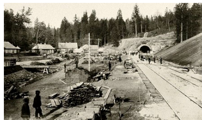
Lietuvos Gelezinkeliai will renovate a railway tunnel built 150 years ago.
